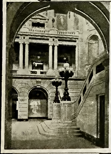
FIRST FLOOR LOOKING ACROSS ROTUNDA.
